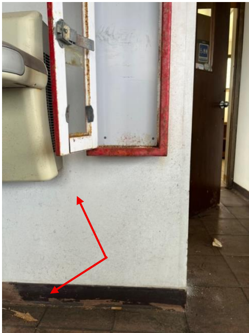
No asbestos detected in covebase or sheetrock/joint compound
