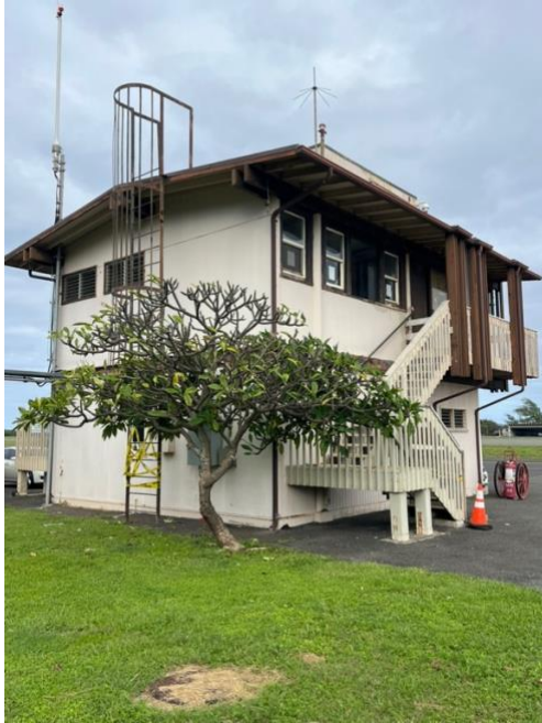
Dillingham Airfield Control Tower Planned for Demolition
