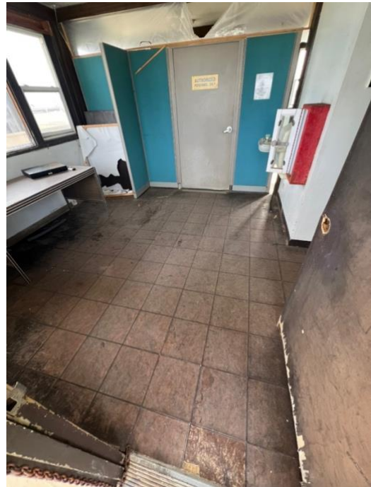
No asbestos detected in brown floor tile
